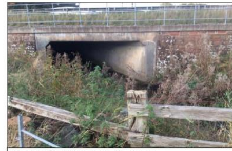
Photo Location 3: Culvert facing downstream
