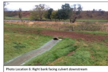
Photo Location 6: Right bank facing culvert downstream
